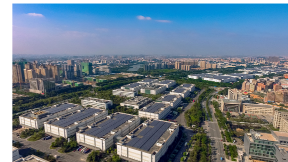
Smart PV plant at Huawei's Southern Factory in Dongguan Capacity: 17.5 MW Connected to the local grid in June 2012
