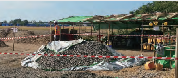
Base station under construction
