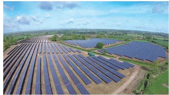
Smart PV plant in the UK
