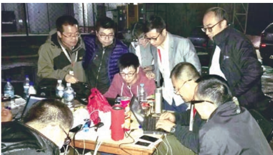
Huawei engineers restoring communications networks in the customer's equipment room
