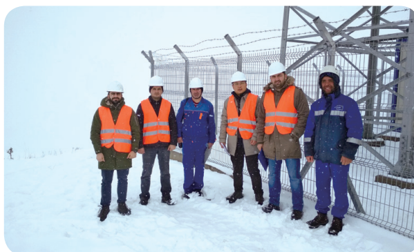
Huawei's service staff and partners check site installation safety (photo taken by Togrul Murtuzayev).
