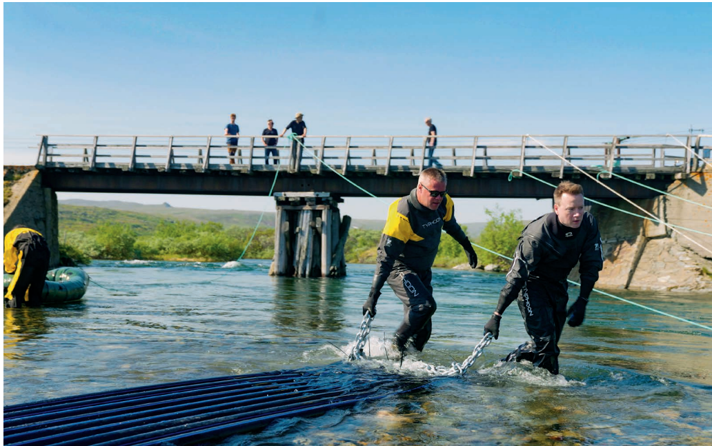
Working with volunteers to install the system (author on the left)
