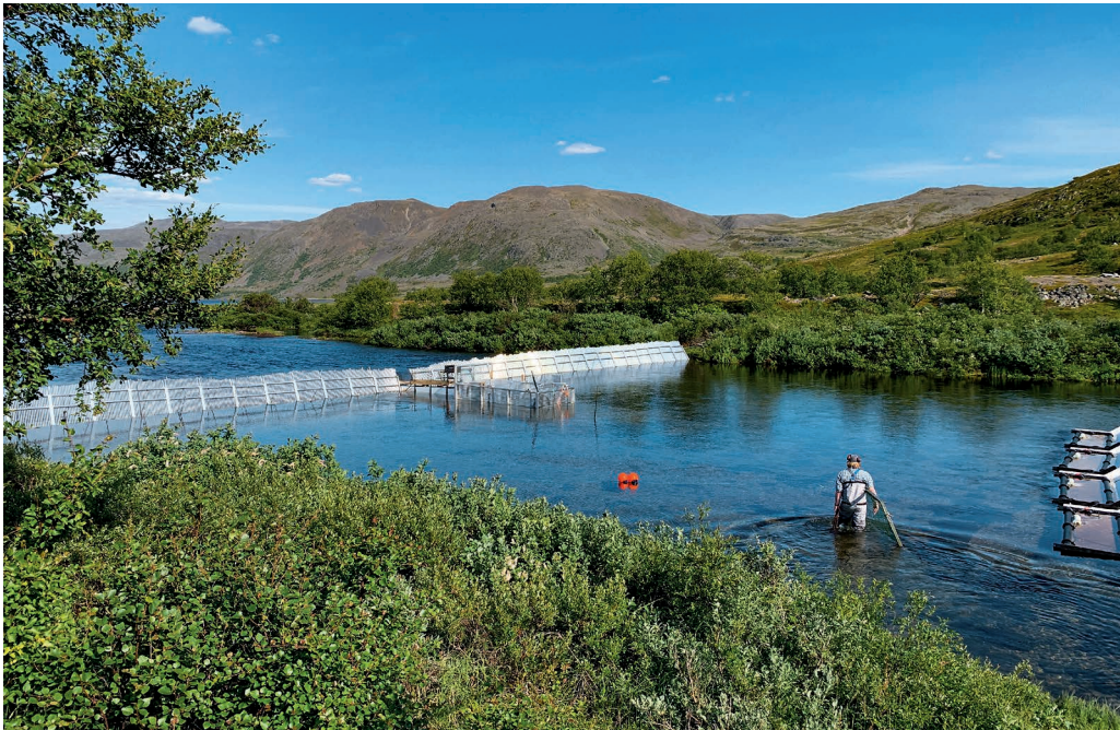
The tunnel filter takes shape in the Storelva River
