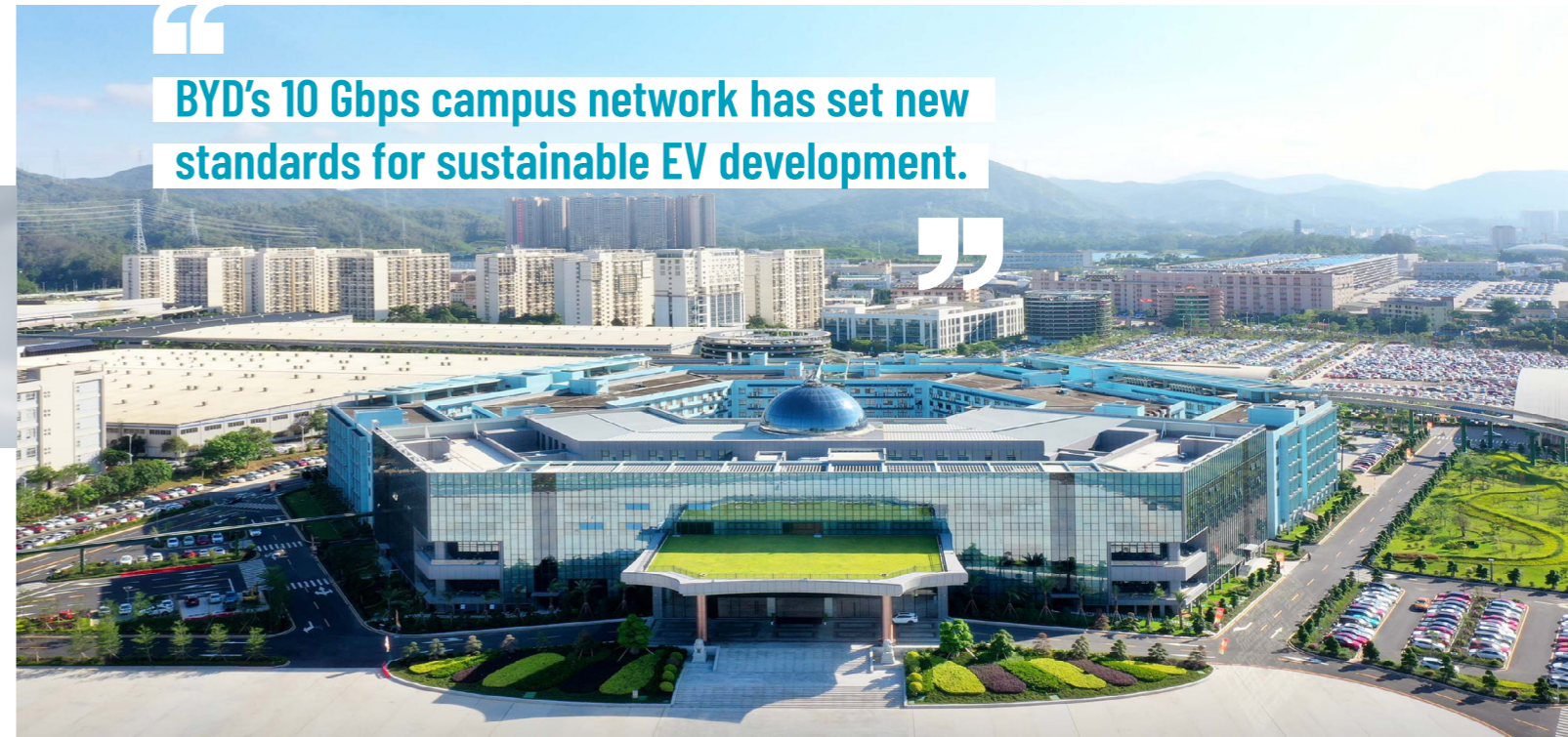
BYD Headquarters in Shenzhen, China
