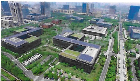
Huawei Hangzhou Research Centre
