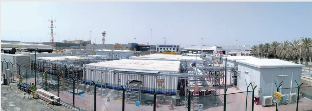
The data center at Dubai Airports
