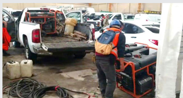
Huawei sends diesel generators to a site to ensure smooth communications
