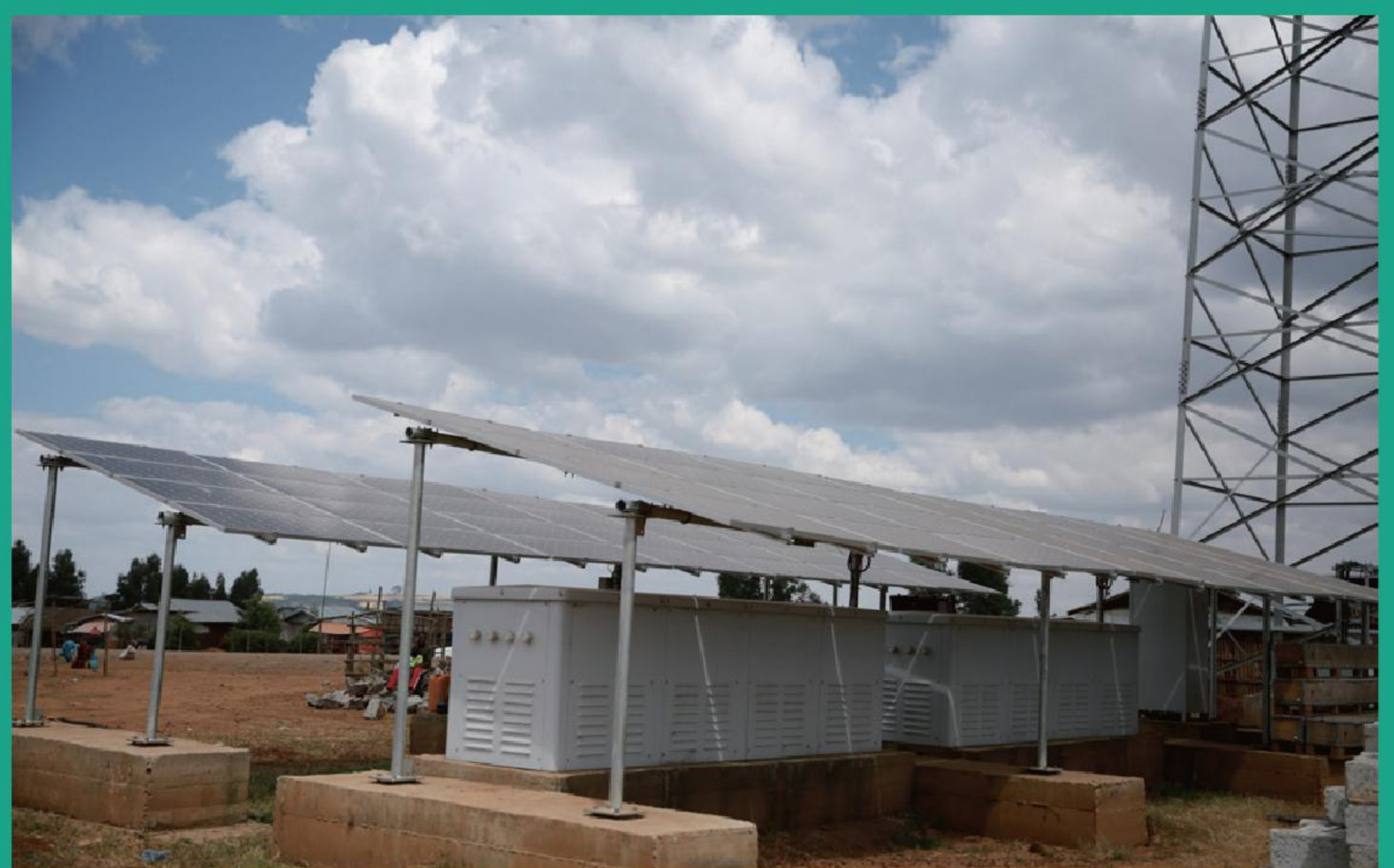
Figure 20 Replacement of diesel generators with PV power in Pakistan
