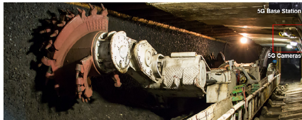
Figure 3: 5G coal mine
